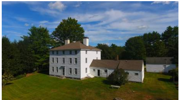
Unique aerial view of the Pownalborough Court House from the side facing the Kennebec River
