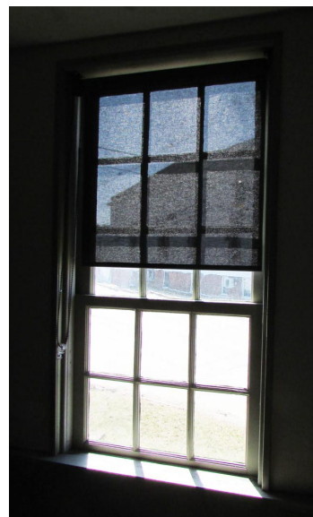
UV shades protect furnishings at Chapman-Hall House
